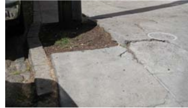
Cracked Sidewalks
